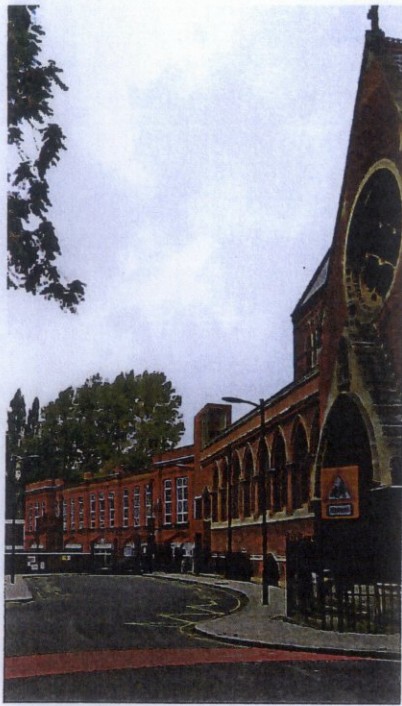
NOVEMBER 2014 Red pigmented concrete facade. Window mullions & lintels red pigmented concrete.
